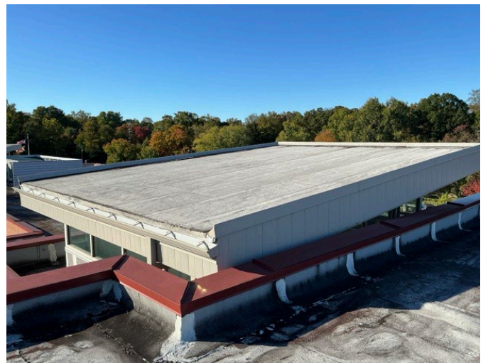
6 - SECONDARY ROOF OVERVIEW
