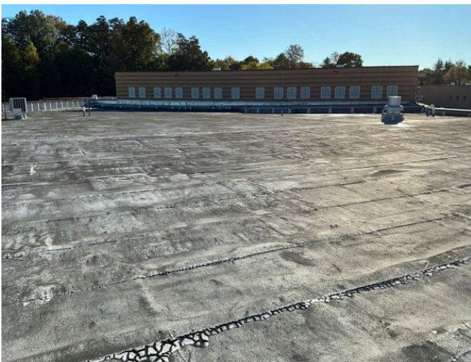
5 - PRIMARY ROOF OVERVIEW
