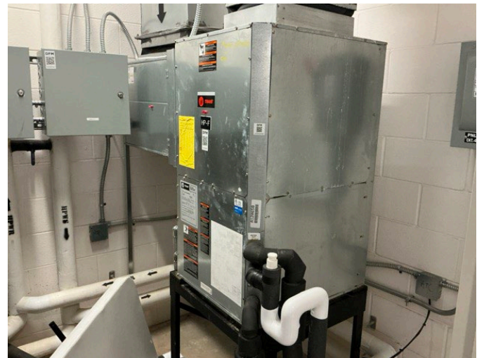
28 - WATER SOURCE HEAT PUMP
