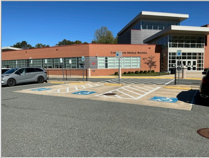
OVERVIEW OF ACCESSIBLE PARKING AREA
