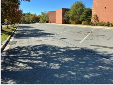
Surface cracks and faded lines - AssetCALC ID: 9956944
